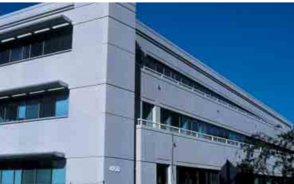
The northeast corner features an obtuse angle that matches the acute angle on the northwest corner, allowing the building to parallel two streets on its irregular site. Precast corner panels wrap around the corner to add to the aesthetics and avoid obvious connecting points.
