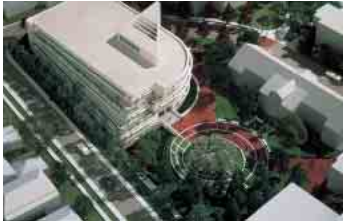
This model of the new patient support services building at the University of California at Davis medical center shows the distinctive offsets of each floor. A wide variety of precast concrete architectural panels were used to create the facade, which includes only one 90-degree corner.
